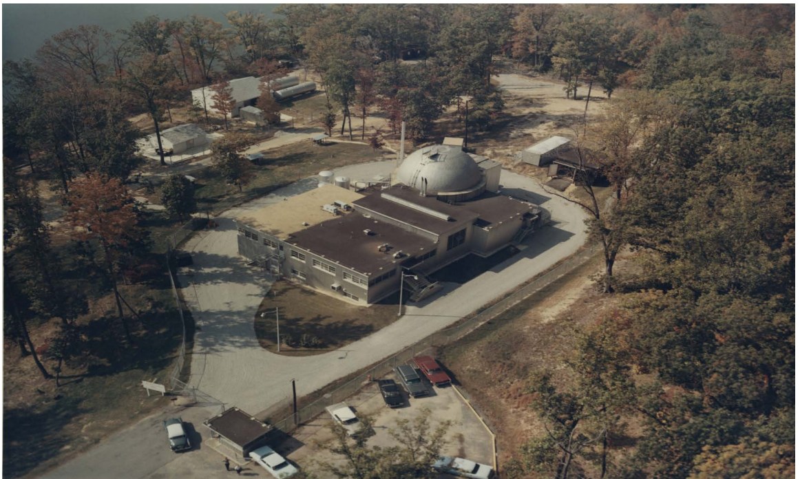
Figure 3: Aerial view of the SM-1 in the 1960's. 8
